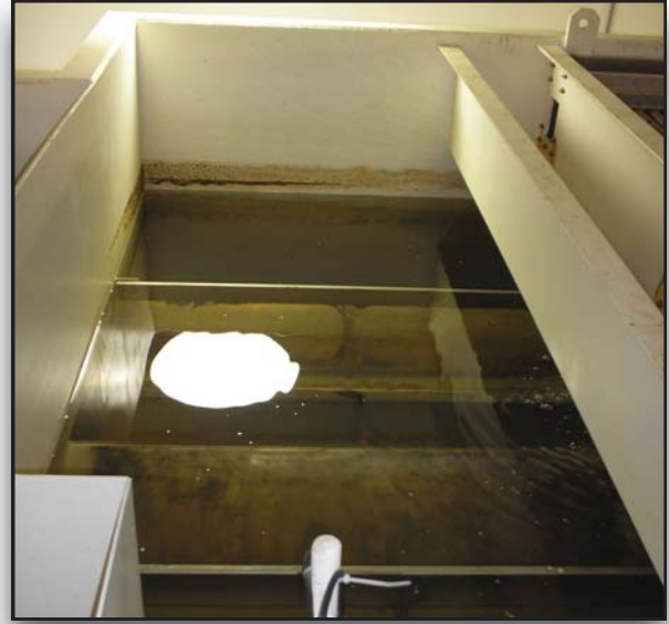
Filter section with Simul-Wash™ trough for sustained combined air/water backwash.
