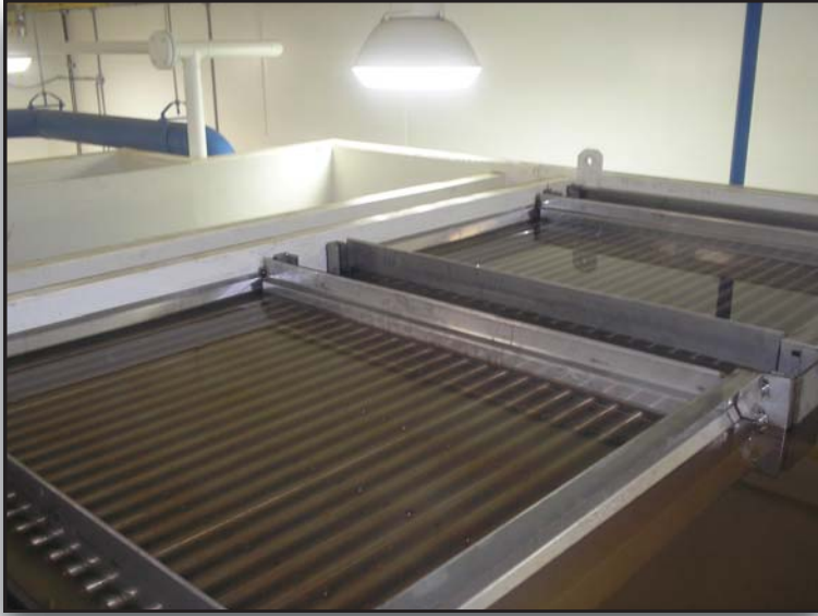
Sedimentation compartment with plate settlers
