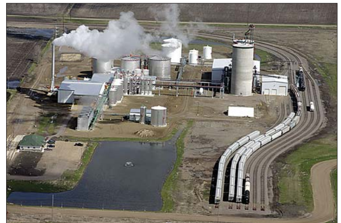
Granite Falls Ethanol Plant
