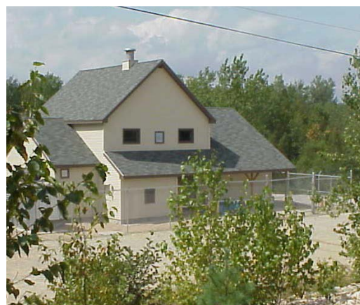
Town of Raymond Water Treatment Plant
